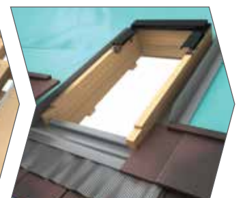
Install roof window
