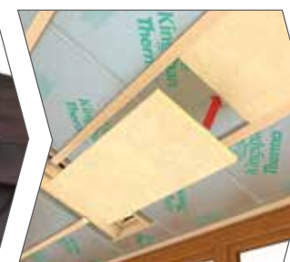
Install insulation between batten
