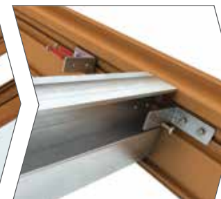
Fix rafters to ring beam
